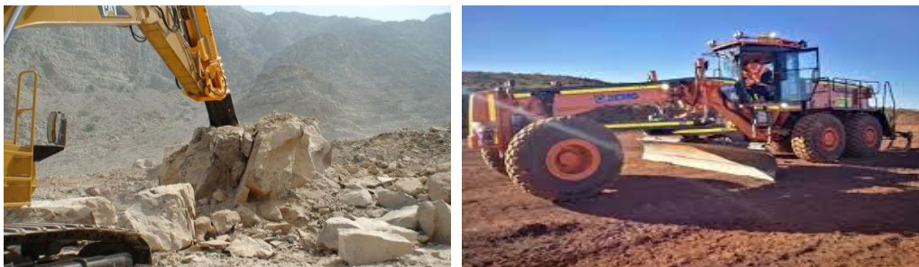
Figure 3.8 Rock Breaker and Road Grader
